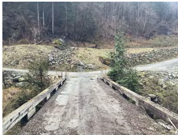
Right bank approach viewing from bridge deck
