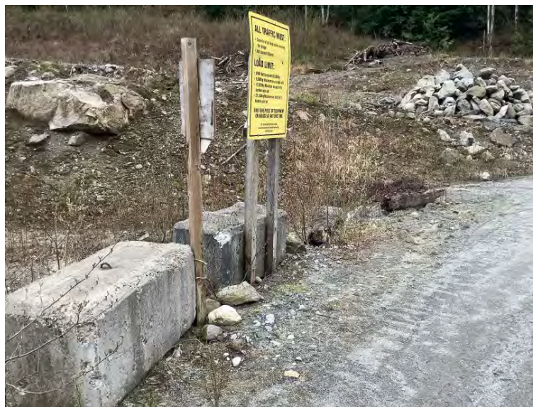
Approach Barrier, left upstream
