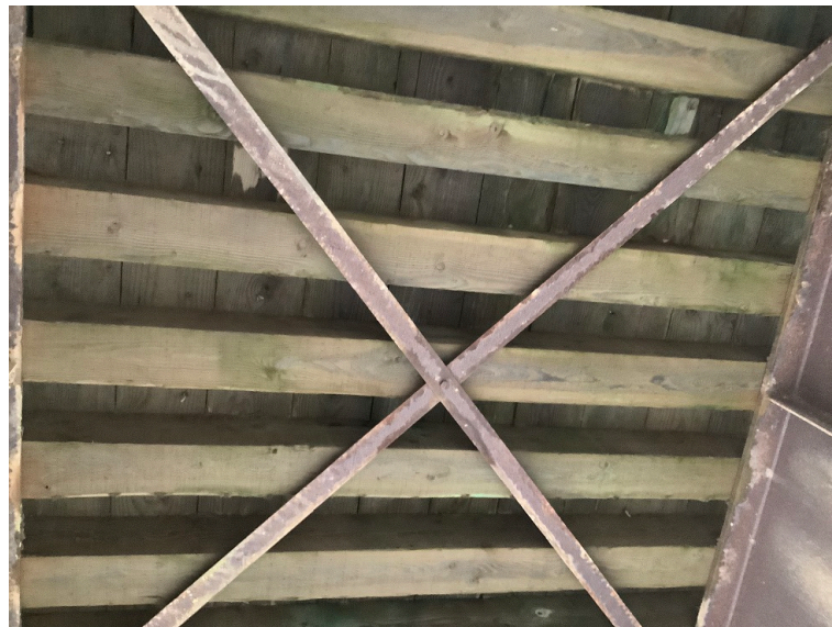
Deck condition from underneath
