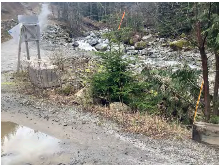
Approach Barrier, right upstream
