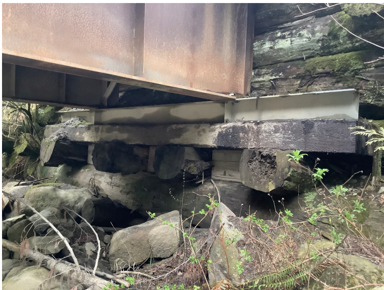
Right Bank Abutment when facing downstream
