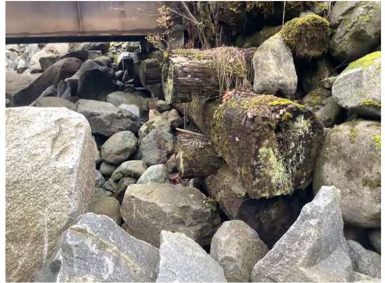
Downstream left crib end
