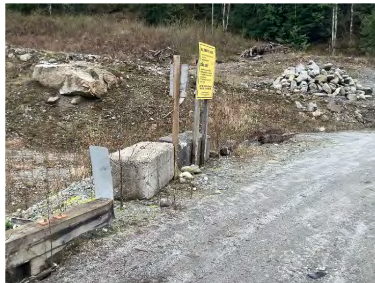
Approach Barrier, left upstream
