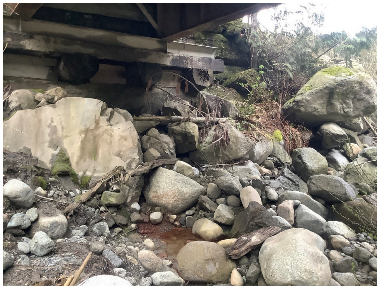
Right Bank Abutment when facing downstream
