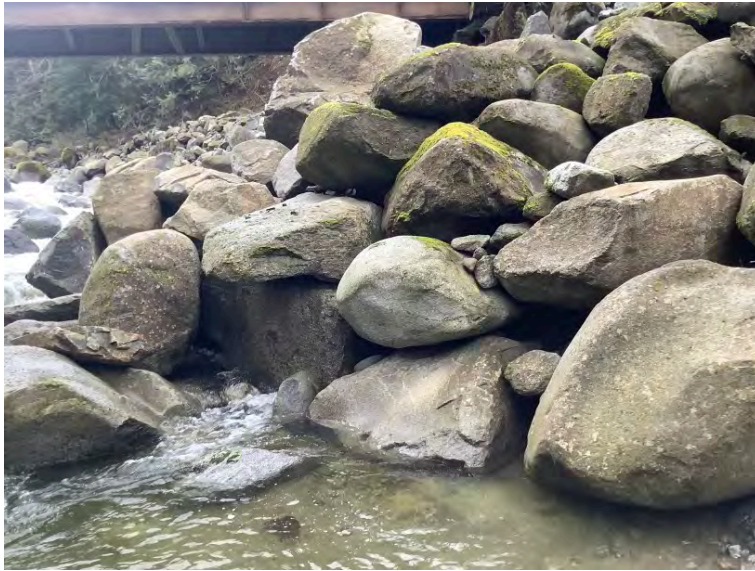
Downstream left riprap toe
