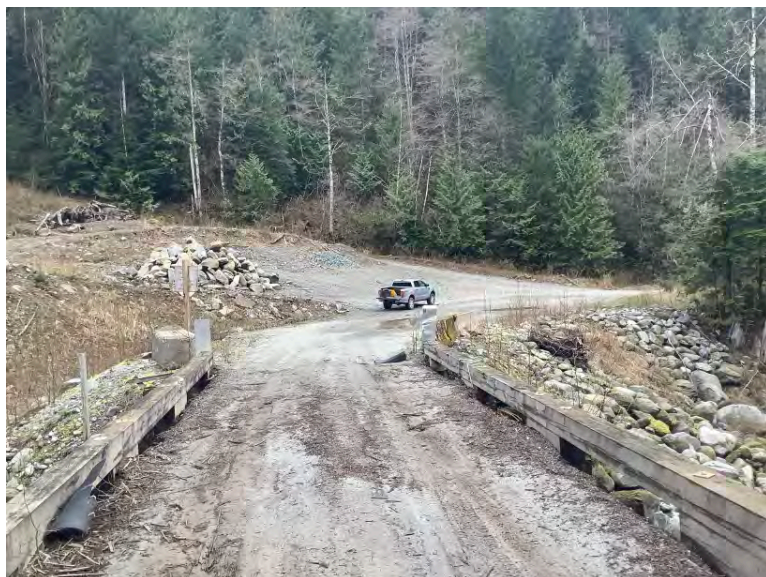
Left bank approach viewing from bridge deck
